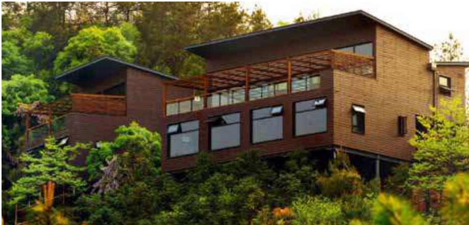
naked Stables Private Reserve is targeting LEED Platinum certification
