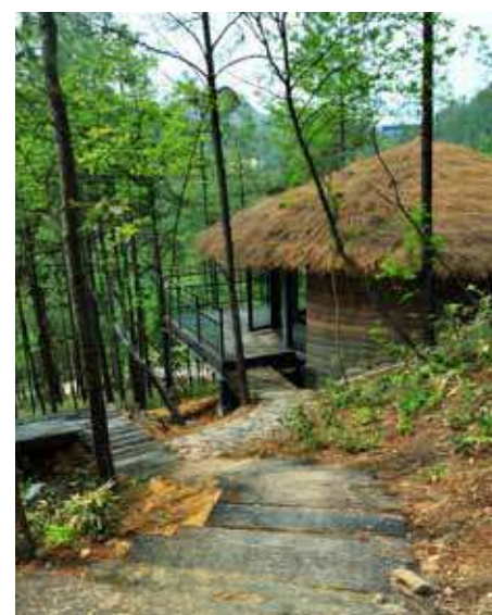
naked Stables Private Reserve highlights traditional building techniques using natural materials such as bamboo
